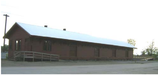
C B & Q Freight House Renovated and Restored
